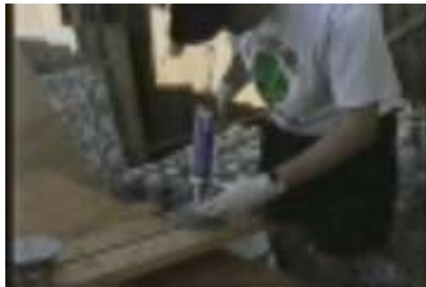
Figure 5 Applying silicone sealant to a pod
